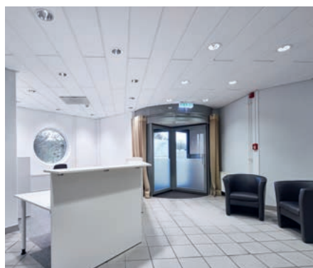
Energy-efficient downlight luminaires at reception.
